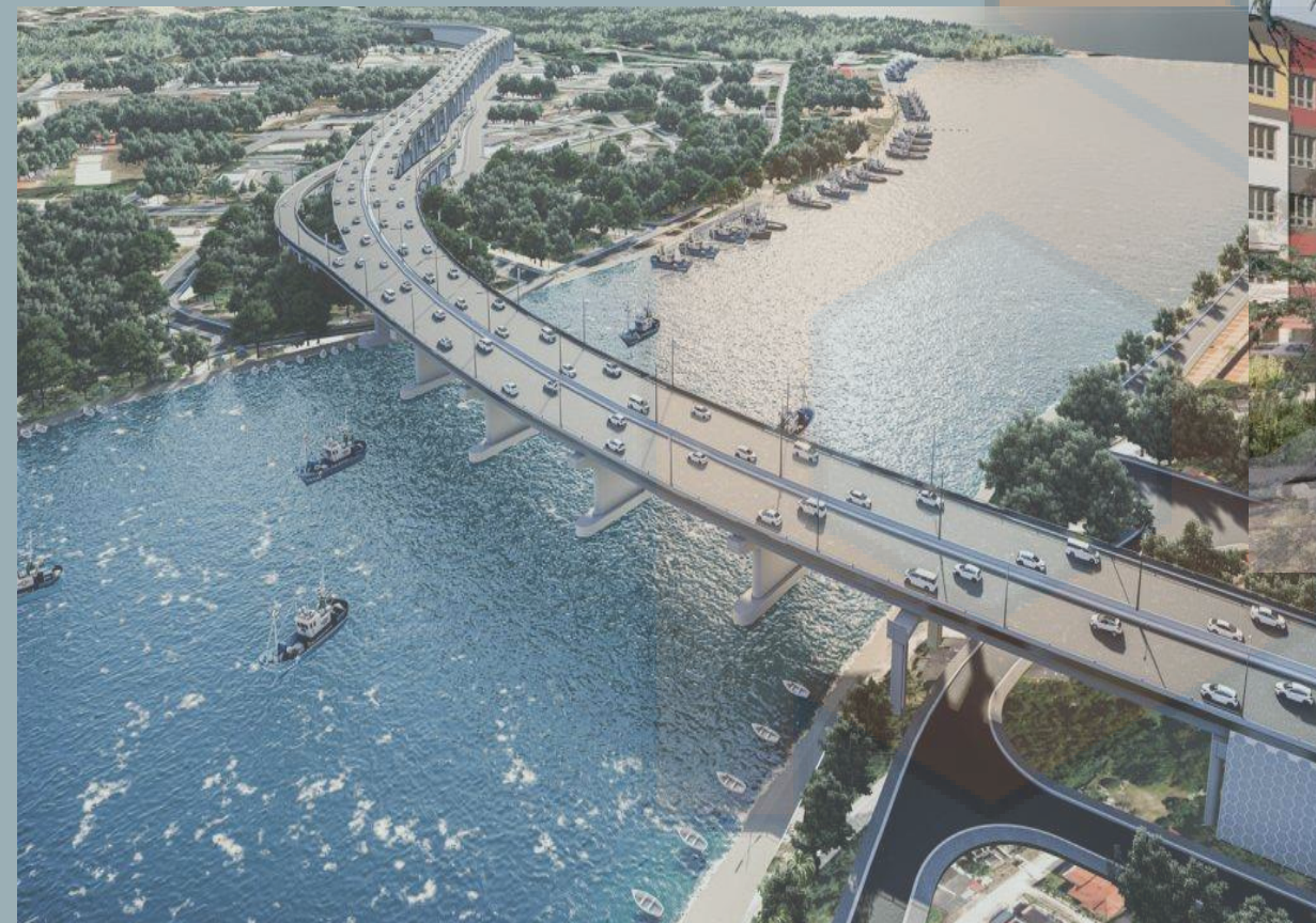
Bridge Cross Over Sg. Marang Contract Value: RM338,500,000.00
